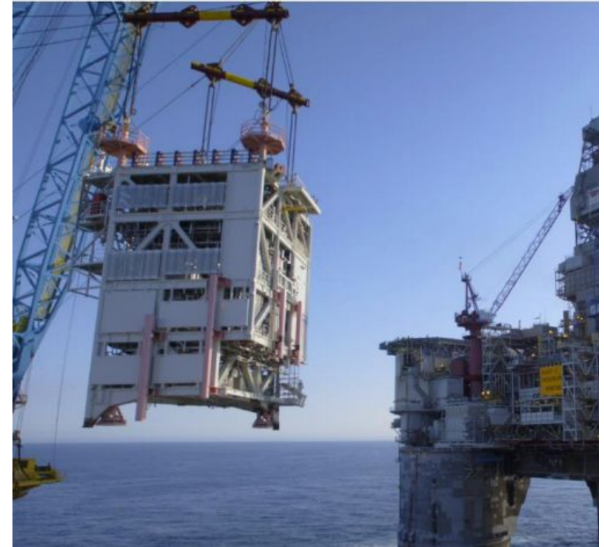
The H25 MEG and Methanol utility module (Dvalin) being lifted towards the Heidrun platform
